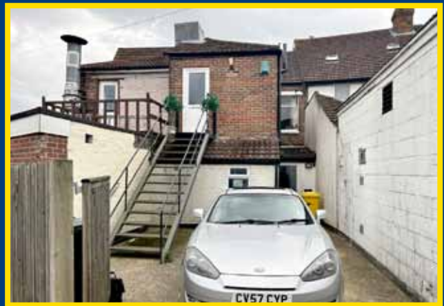
Rear Car Parking Area/Access to Flat
