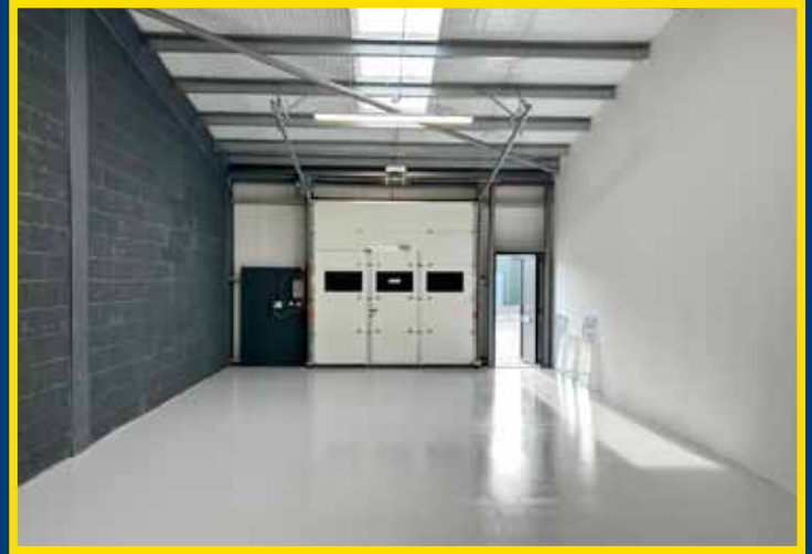
Internal once refurbished
