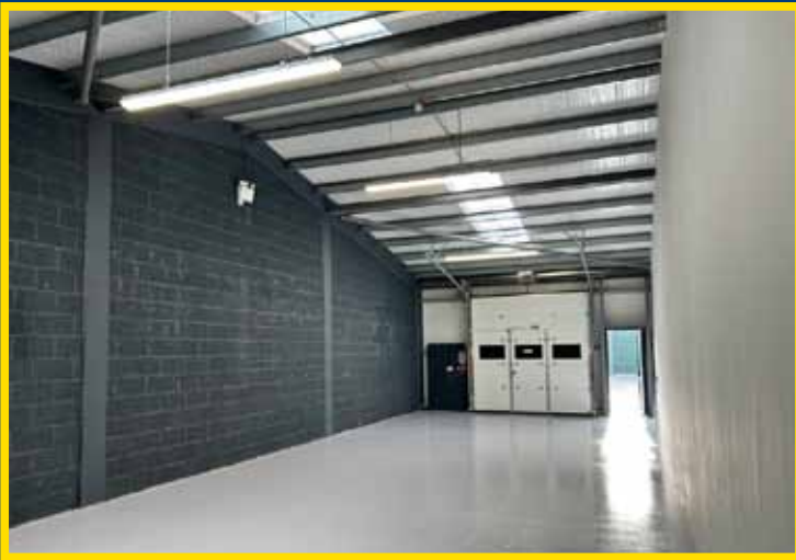
Internal once refurbished
