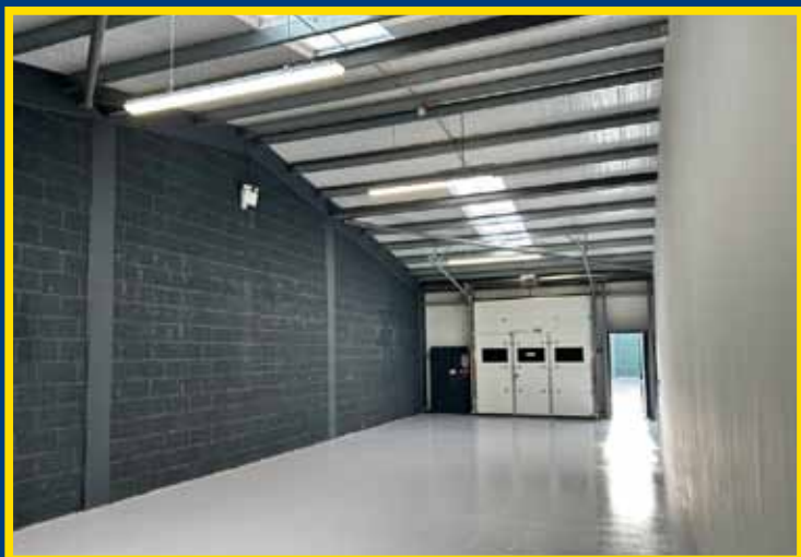
Internal once refurbished
