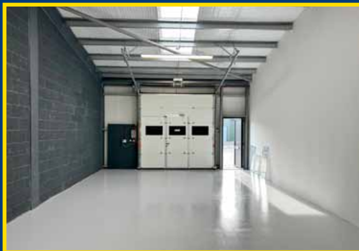
Internal once refurbished
